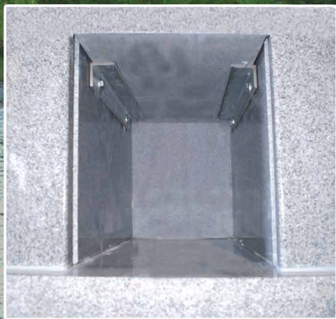
Interior Niche with Door Removed.
